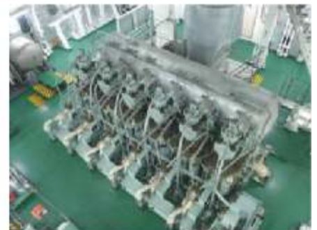
Main Engine Inspection
