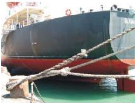
Condition Survey, Hull Inspection
