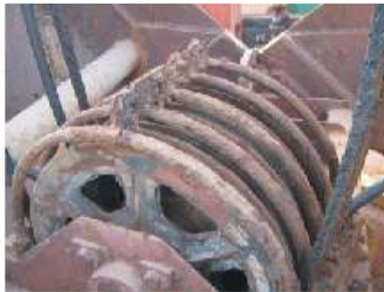
Inspection of runner wire block
