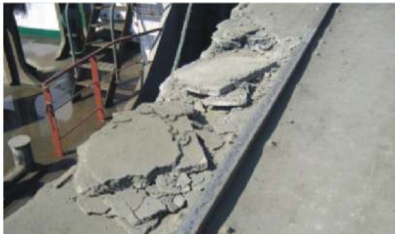
Jetty Damage Survey/Inspection
